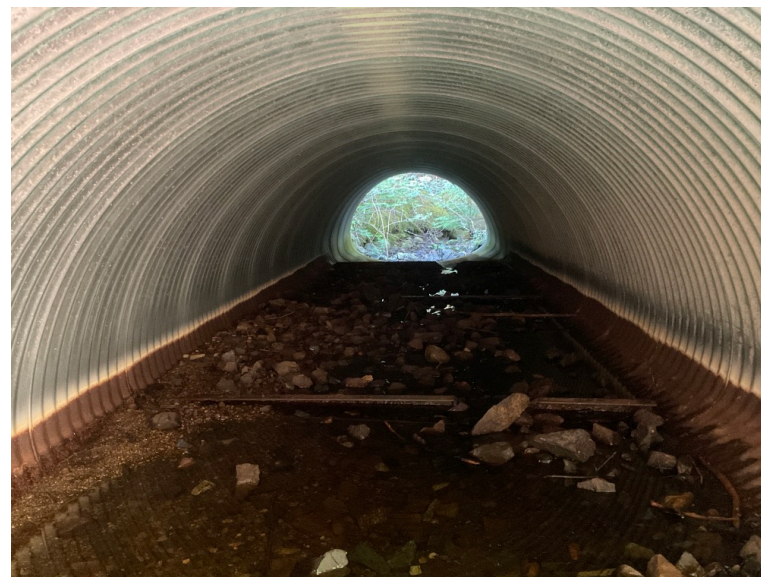
Looking Downstream Through CMP
